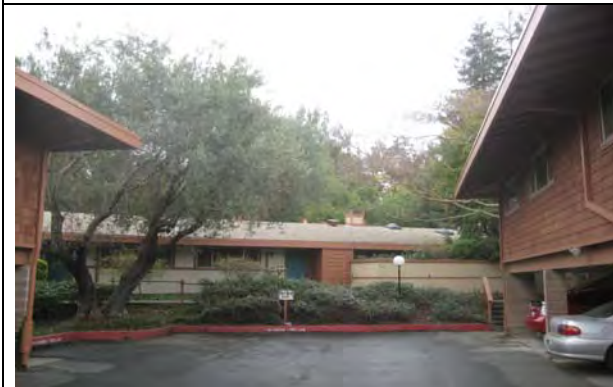
ST-11: Equivalent to apartments adjoining SR 85 along Alice Avenue.
