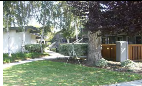
ST-17: Rear yard of 877 Heatherstone - Heatherstone Apartments.
