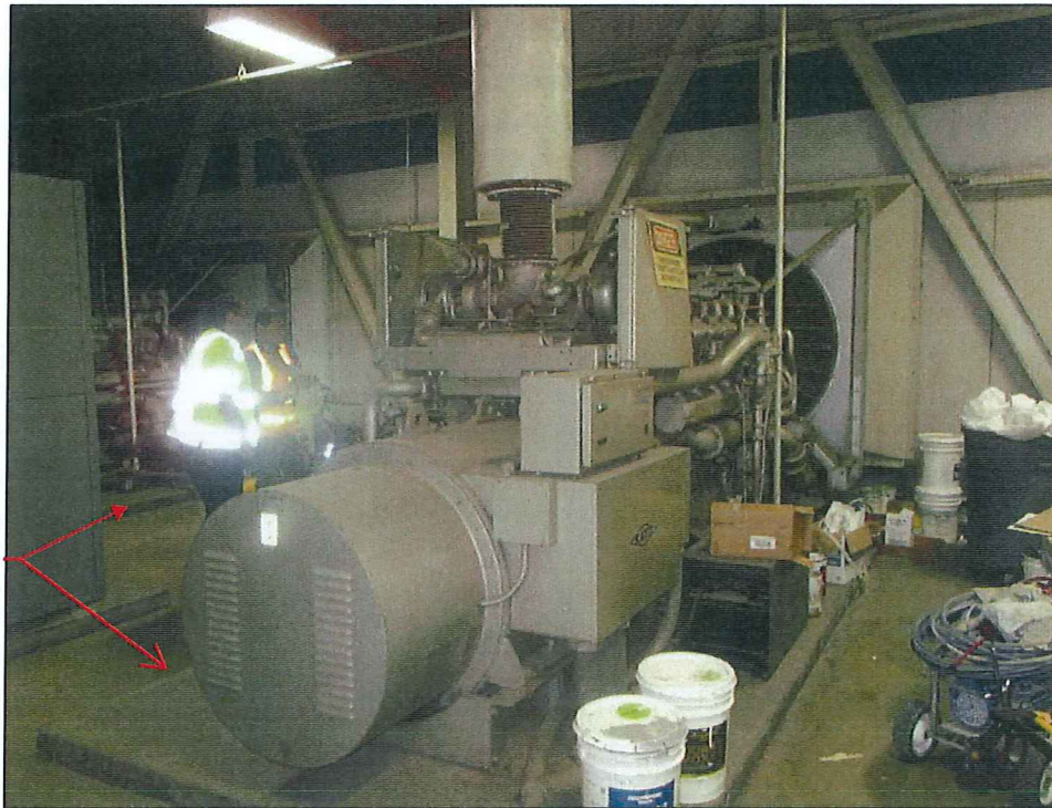
Photograph 19: Gray Concrete Pads- Diesel Generators
