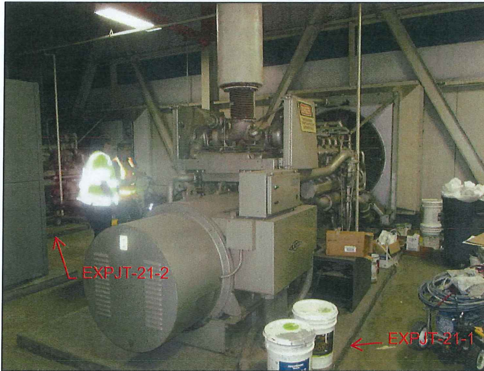
Photo 17: Expansion Joints Caulking
