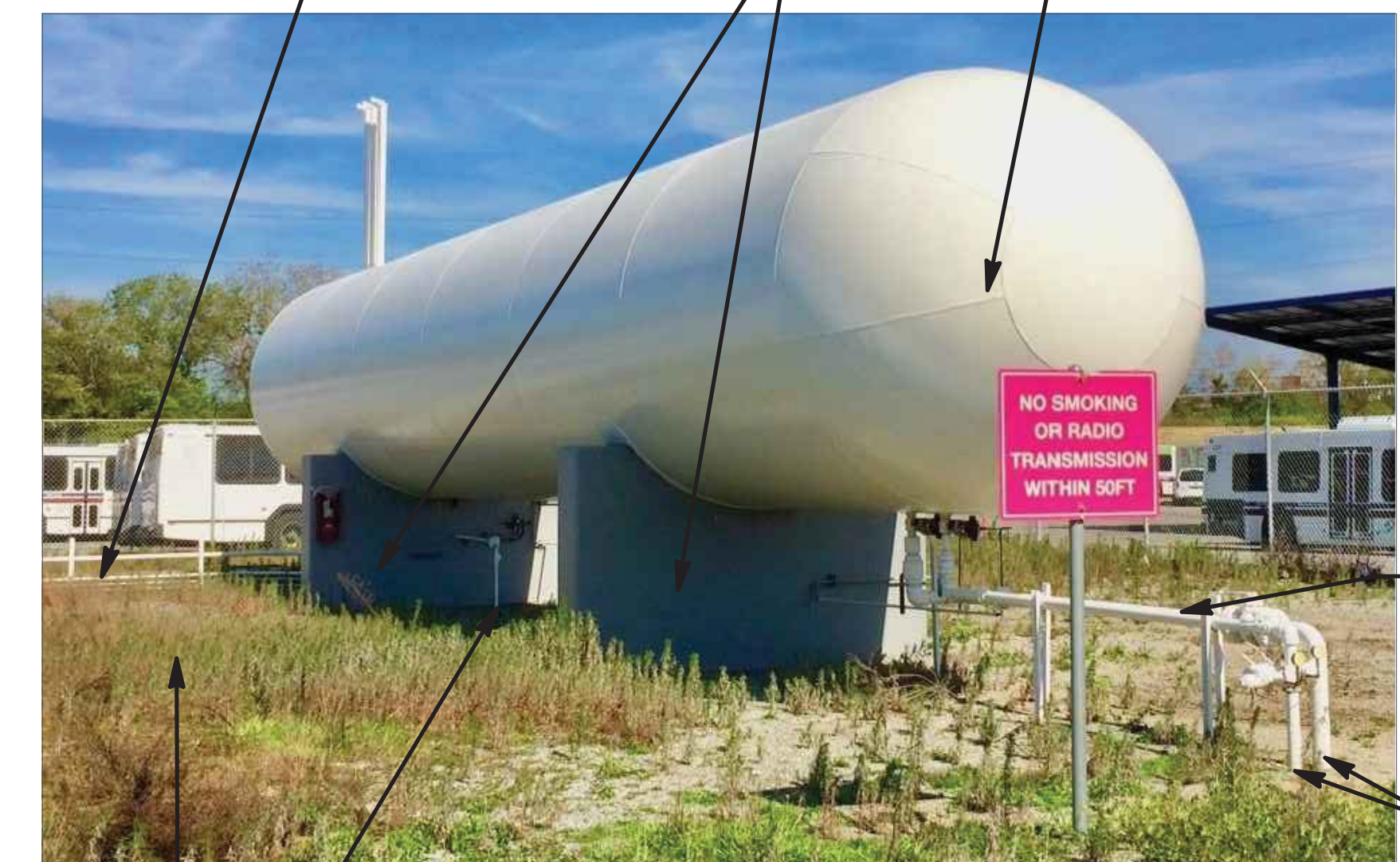
3 30,000 GALLON LPG TANK D3 NTS
