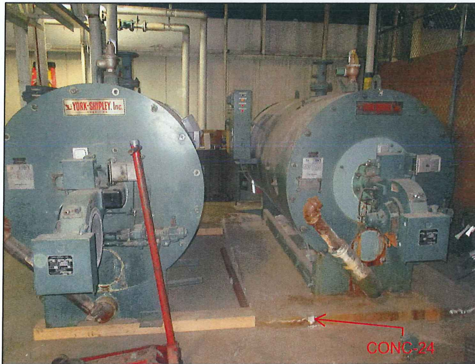
Photograph 18: Boiler Gray Concrete Pads.
