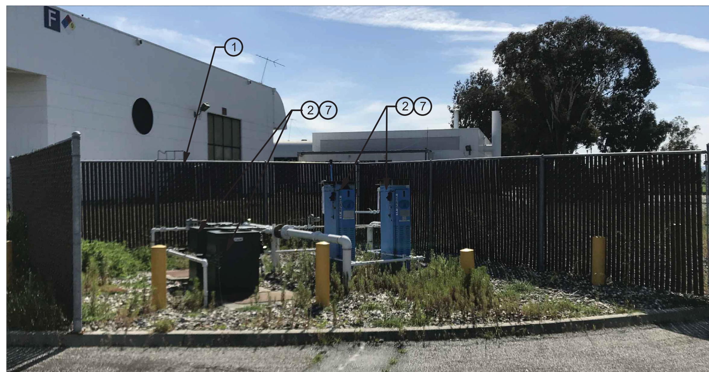
1 LPG VAPORIZERS D3 NTS
