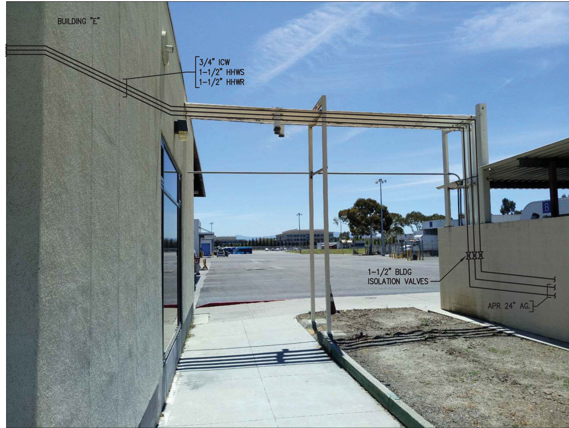
3 HHW & ICW PIPE ROUTING TO BLDG E - NTS
