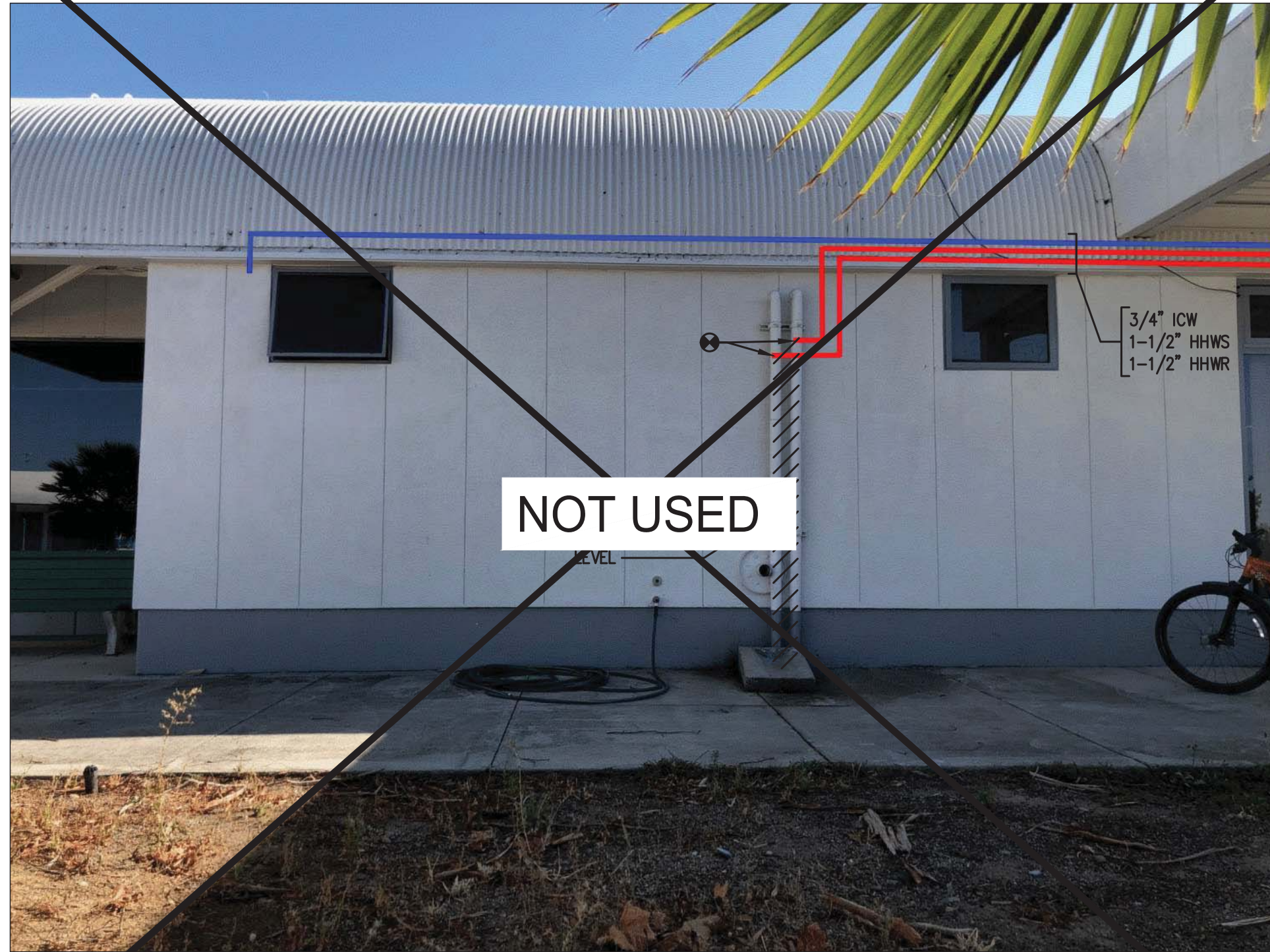
5 HHW & ICW PIPE ROUTING AT BLDG E - NTS
