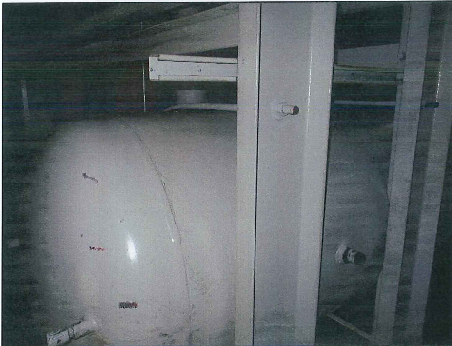
Photograph 10: Expansion Tanks/Brackets
