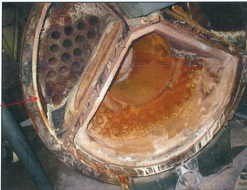
Photograph 8: Boiler Insulation Sampling
