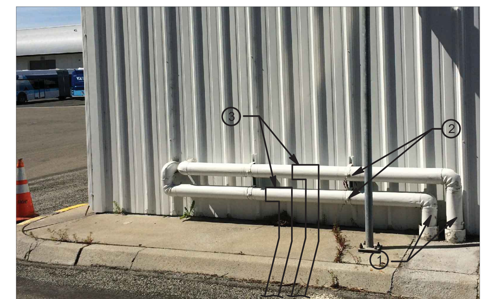
① HWS/HWR OUTSIDE PENETRATION D4 NTS
