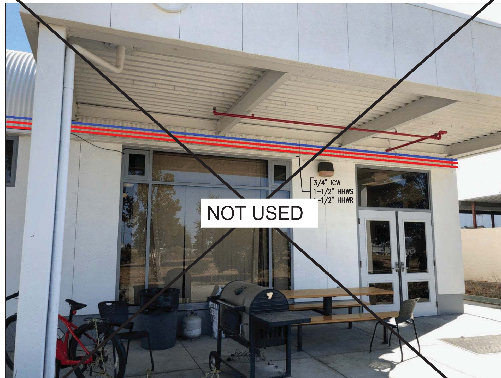
4 HHW & ICW PIPE ROUTING AT BLDG E - NTS
